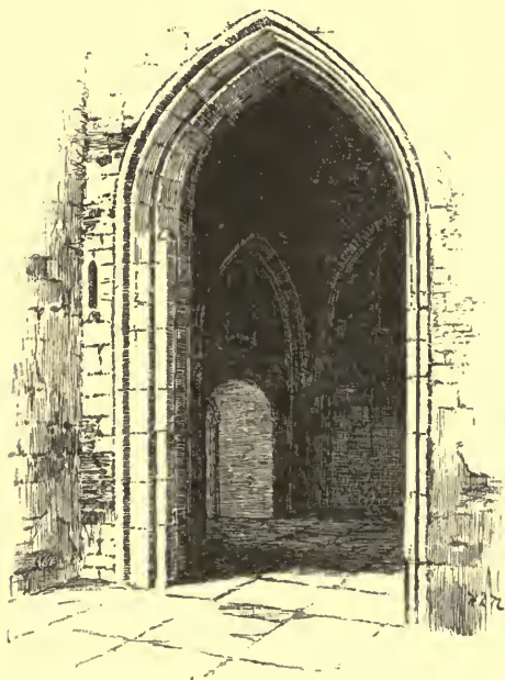
INTERIOR OF PORCH OF THE PARISH CHURCH OF ST. ALPHEGE, LONDON WALL, FORMERLY THE CHAPEL OF THE PRIORY OF ST. ELSYNGE SPITAL
